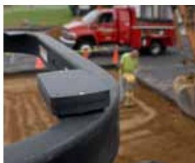
Tracker installed on metal frame of roller.
