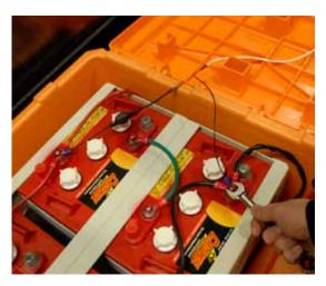
When maintenance is completed, reconnect the tracker's power wires to the battery terminal first
